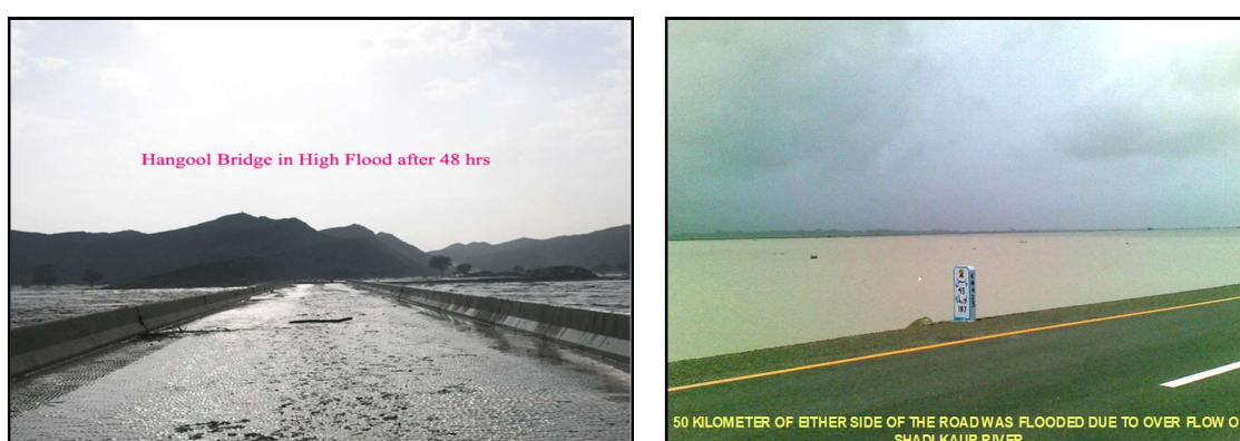
Figure 4-3: Flood Water Inundating the Makran Coastal Highway N-10
